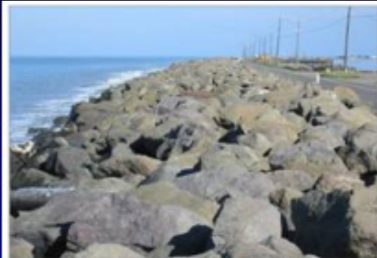
Riprap on Ediz Hook in Port Angeles
