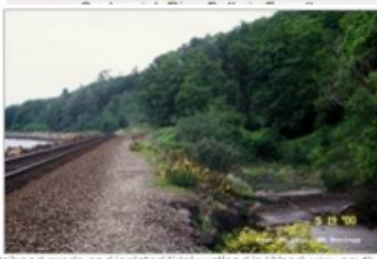
Railroad grade and isolated tidal wetland in Woodway, south of
